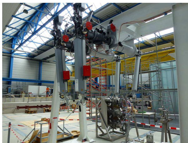
Figure 4: Hot-Cell mock-up mounted on the ESR roof
