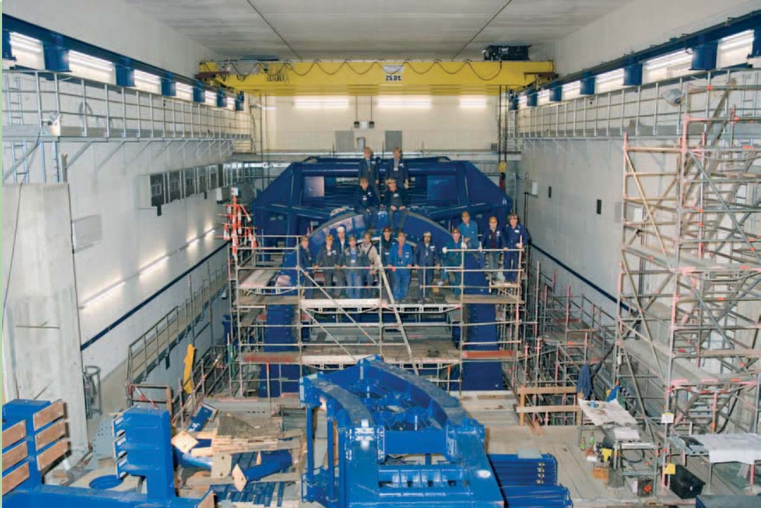
The gantry room during the assembling of the gantry structures.
