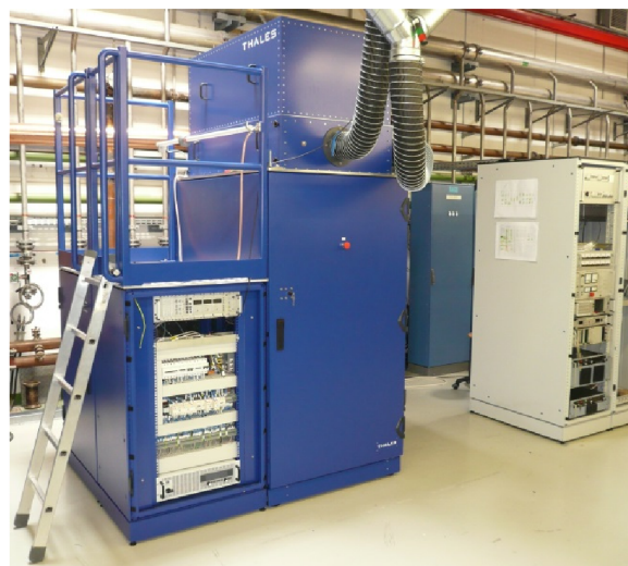
Figure 2: New 1.8 MW high power cavity amplifier prototype installed at the UNILAC RF gallery plus control rack equipped with grid power supplies, new measurement & fast interlock unit, and further control elements.
