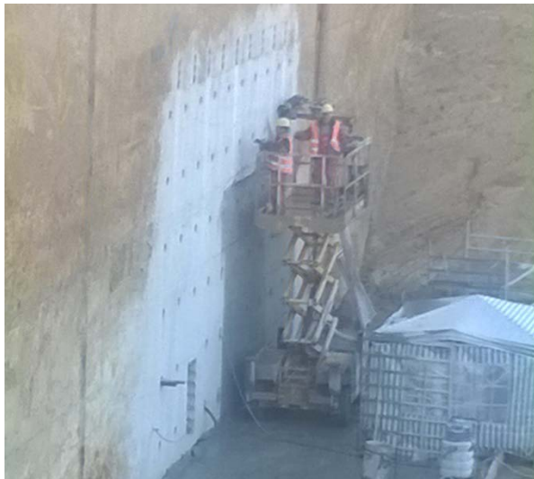
Figure 2: Construction Area of GAF: wall of existing hall is opened to connect new beam line tunnel towards FAIR.
