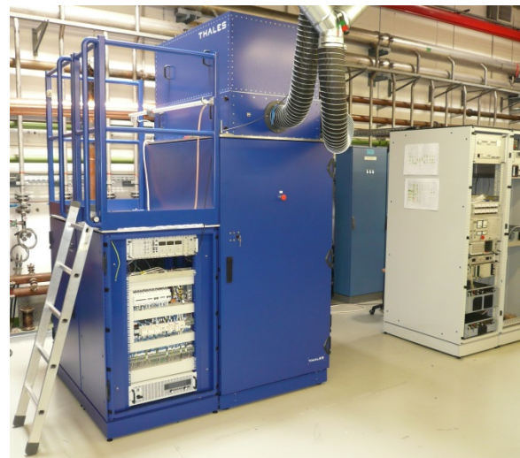
Figure 2: New 1.8 MW high power cavity amplifier prototype installed at the UNILAC RF gallery plus control rack equipped with grid power supplies, new measurement & fast interlock unit, and further control elements.
