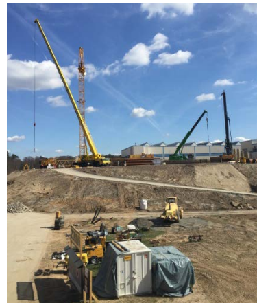
Figure 2: The soil shielding on top of the SIS18 tunnel is presently enhanced. This requires a table like construction, carrying the additional weight on top of the existing tunnel.
