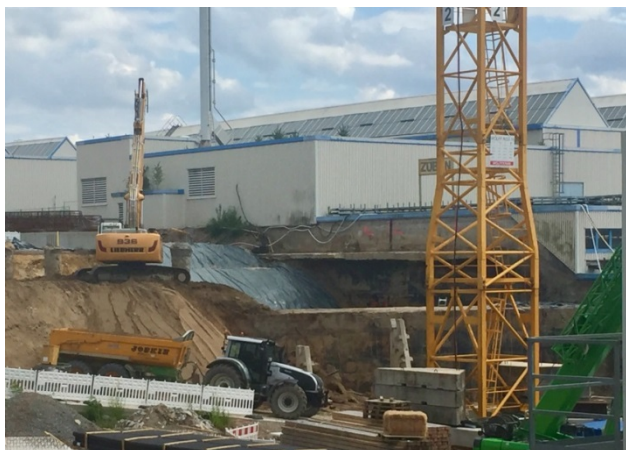
Figure 2: Construction works for the interface of the Proton Linac building
