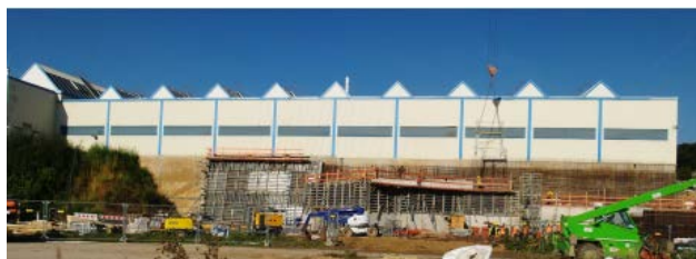
Figure 3: Construction works for the interface to the FAIR tunnel 101.
