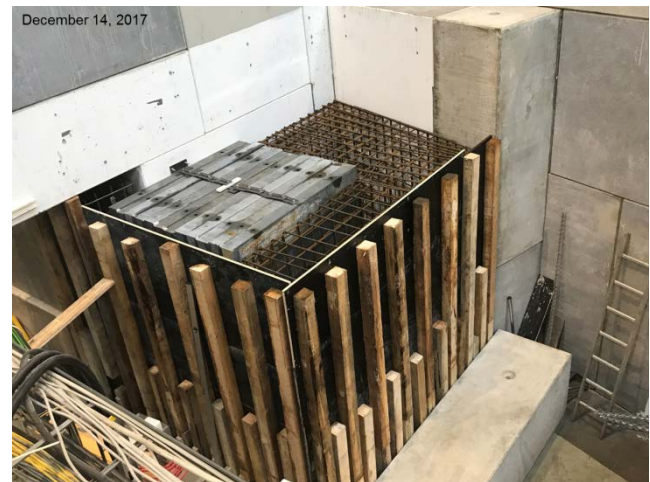
Figure 6: The Iron core of the beam dump is prepared for concrete pouring.
