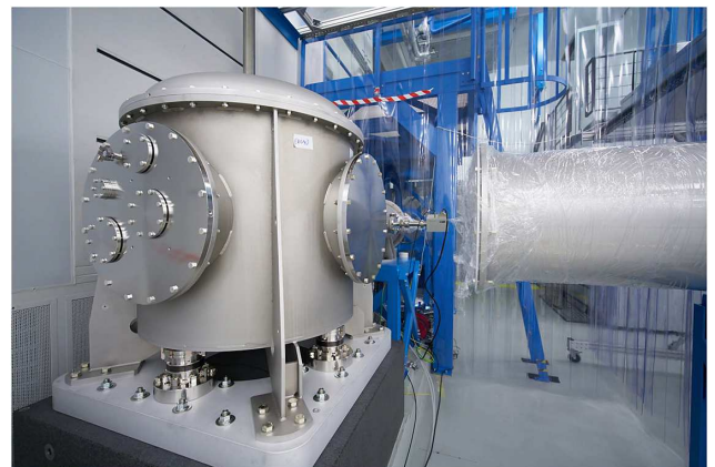
Figure 22. Clean installation in experimental hall E3. Local cleanroom tents were constructed and built to allow clean access to the mirror chambers and to connect them via bellows to the adjacent DN500 pipes.
