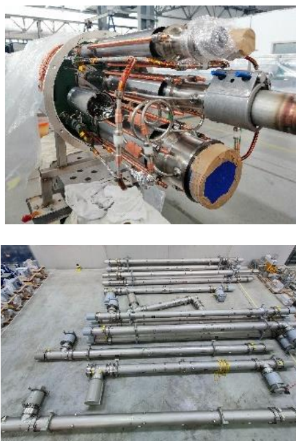
Figure 4: Cryogenic bypass lines containing the LHe process lines and the four main magnet bus bar systems made of Nuklotron type cable.
