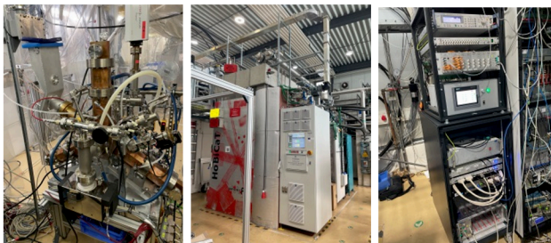
Figure 7: a) Cavity, b) Solid State Amplifier, and c) Controls and Digital LLRF.
