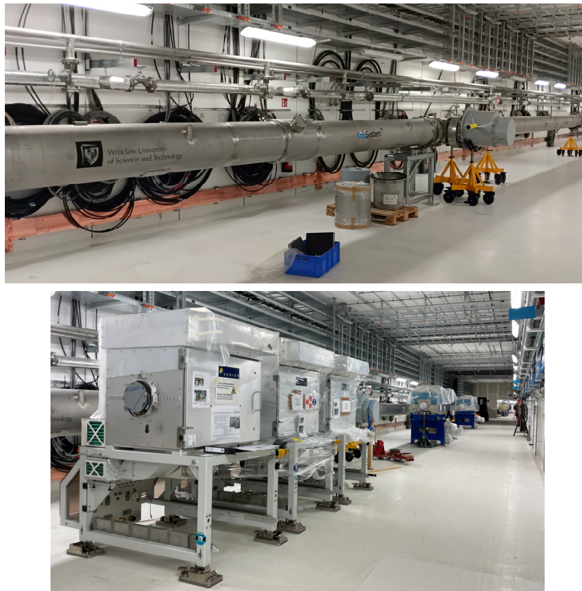
Figure 6. Installation of the by-pass line at semi-final position on temporary supports (top); installation of accelerator components-room temperature cavities- in front of the line (bottom)
